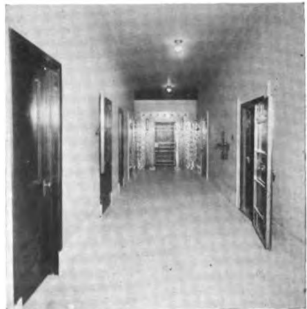
MAIN VAULT CORRIDOR
